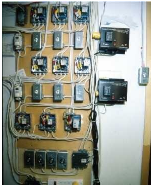
Wiring your own grow room is relatively easy. This grower hardwired a separate breaker box and timer that supports four lamps.
