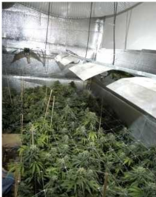
Avoid long, unnecessary ducting such as shown above. Keep ducting as short as possible.
