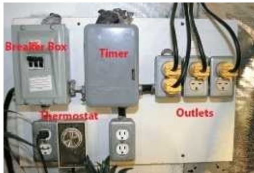
Wiring your own grow room is relatively easy. This grower hardwired a separate breaker box and timer that supports four lamps.
